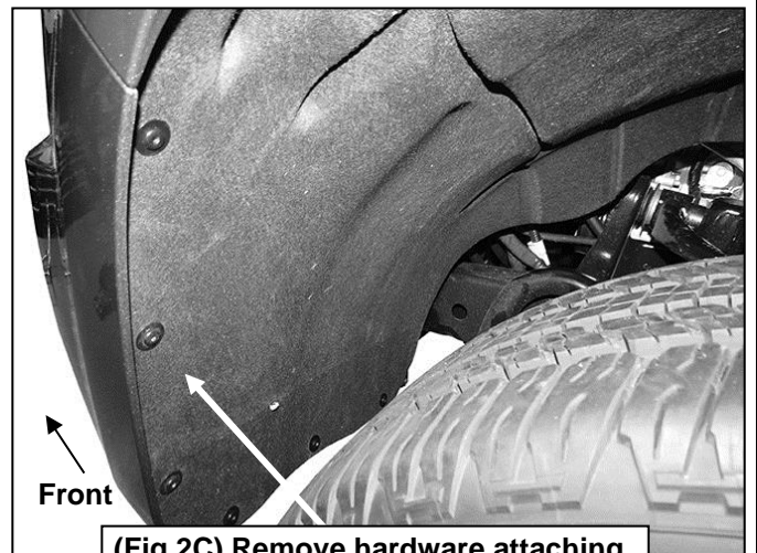
(Fig 2C) Remove hardware attaching fender liner to bumper cover
