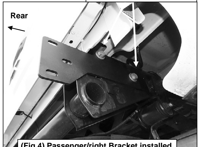
(Fig 4) Passenger/right Bracket installed
